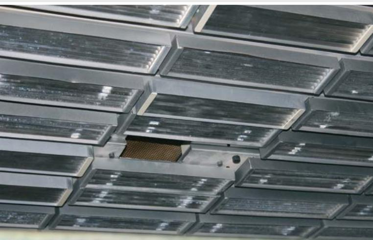
*Heating field comprising radiant heaters, arranged in columns and rows. One heating field was removed for the viewing field of the camera.*
